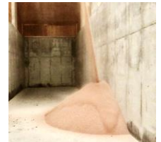
First load of potash into the new plant
